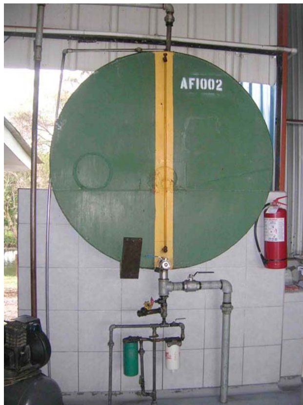
Pic 12: After quality control the bio-diesel is stored in these green tanks ready for distribution
